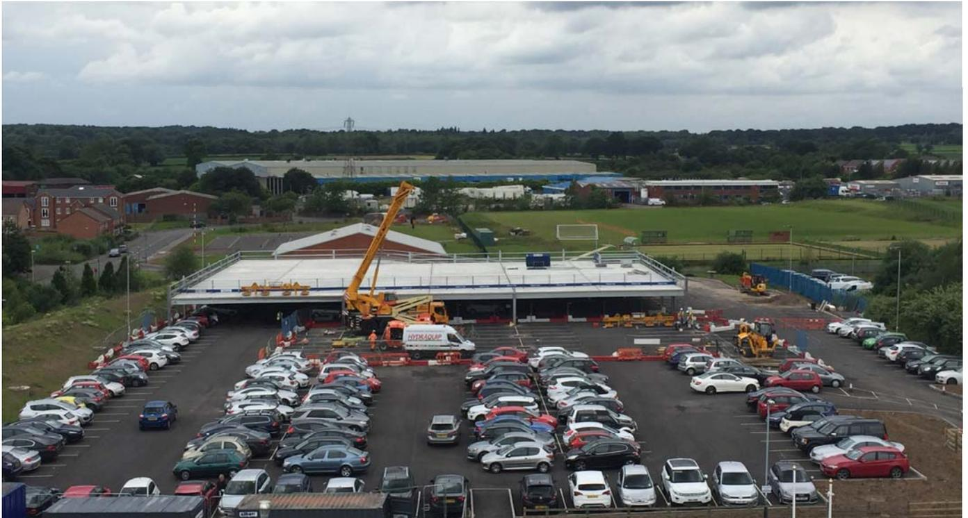
The erection of the car park (above) took strict logistics management to ensure that the 200 staff cars could still access the existing ground floor car park. Now completed (below) the additional spaces will provide additional parking as new staff enter the Head Office extension.
